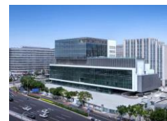
Beijing New View Garden Commercial Centre
